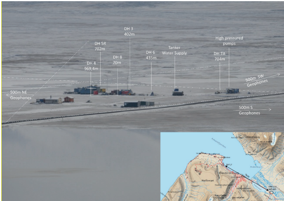
Figure 2. Overview of the UNIS CO 2 Lab well park in Adventdalen, south-east of Longyearbyen. The inset map shows the UNIS CO 2 Lab well park location, as well as the location of the DH1 and DH2 boreholes near Longyearbyen airport. All publications in this appendix are partly based on data from these boreholes. The numbers beneath the well numbers indicate s total drilled depth (TD) of each borehole. All wells apart from DH3 are now plugged and abandoned (P&A). In addition, temporary shallow geophones were installed within a 1 km radius of the UNIS CO 2 Lab well park during the operational phase. Stippled lines shows position for some of the conventional 2D seismic lines acquired in this area.
